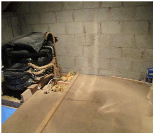
floor space of Attic.
